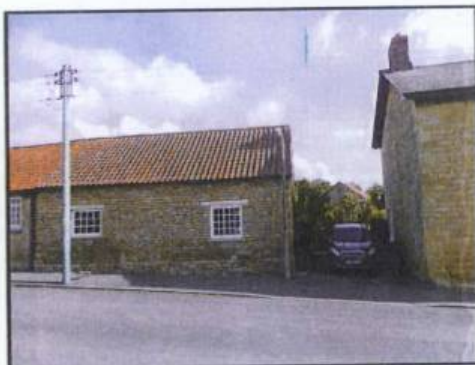
11.2 View of East elevation
